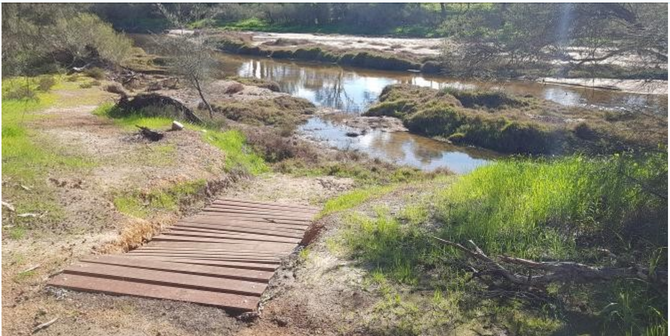
Above: Launching Ramp for kayaks at Weatherall Pool, West Toodyay. The ramp will assist in protecting the river bank, particularly during the Avon Descent.
